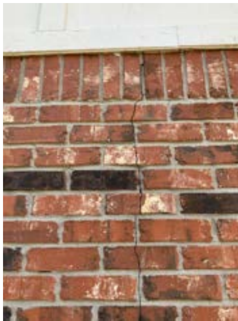
Exterior Southeast Wall (Primary Bedroom)
