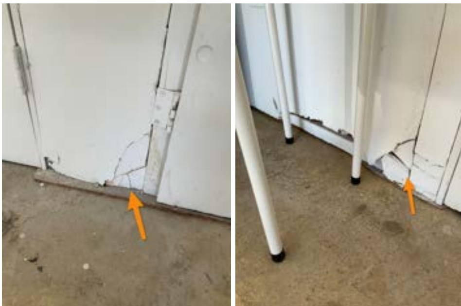
Damaged Drywall
