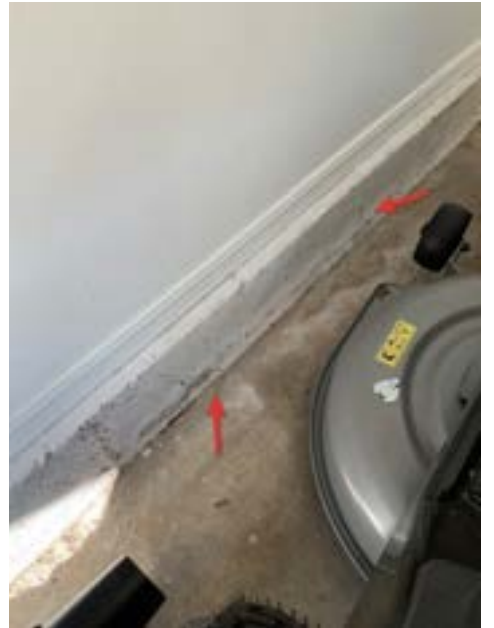
Foundation Cracking
