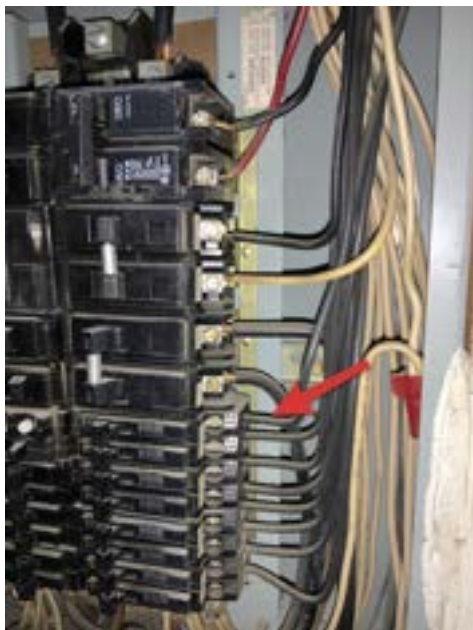
Aluminum Wiring
