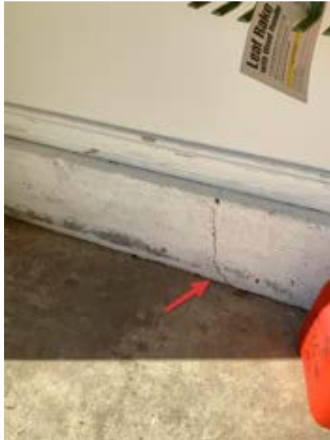
Foundation Cracking
