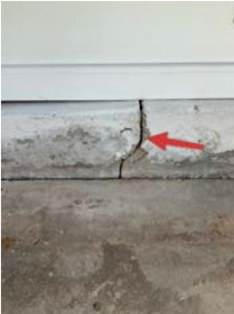
Foundation Cracking
