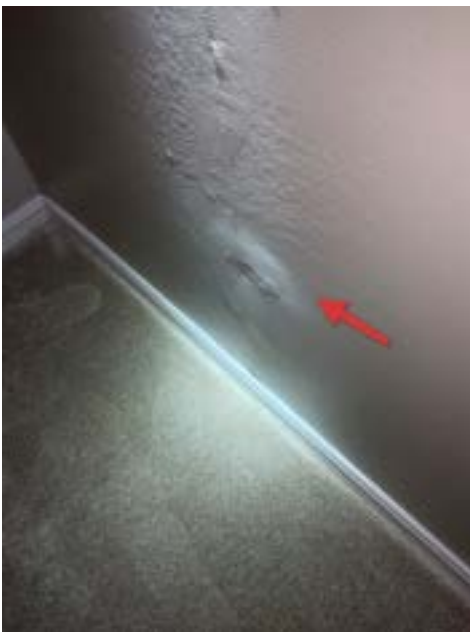
Primary Bedroom- South Wall
