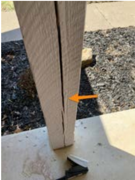
Cracked/Damaged Post
