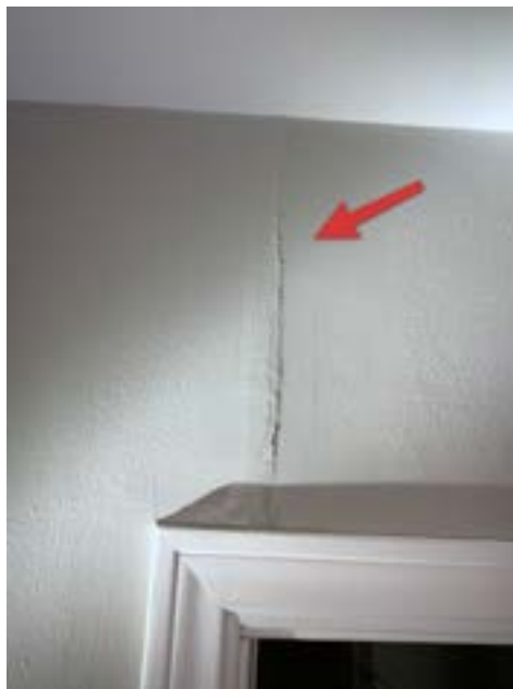
Primary Bedroom-Bathroom Door
