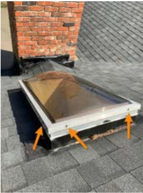
Rusting Fasteners
