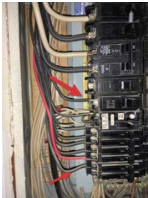
Aluminum Wiring
