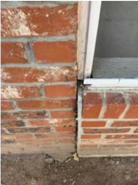
Exterior East (Covered Porch)
