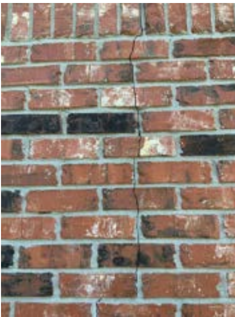
Exterior Southeast Wall (Primary Bedroom)
