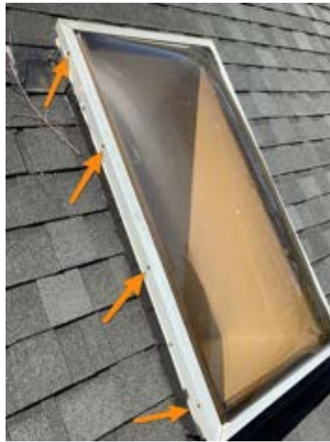
Rusting Fasteners
