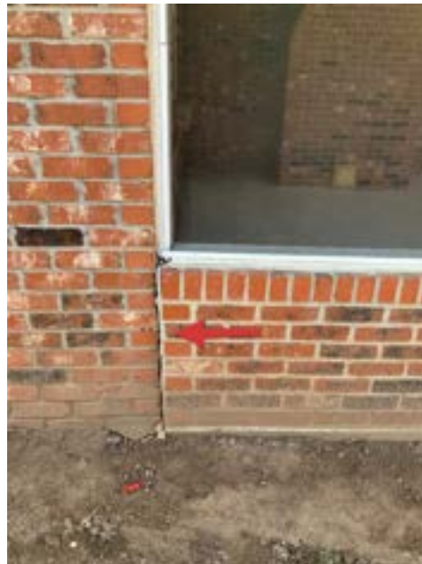
Exterior East (Covered Porch)
