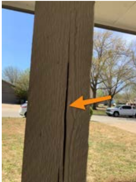
Cracked/Damaged Post
