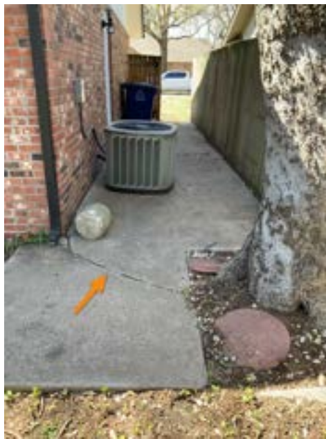
Exterior Northeast Walkway
