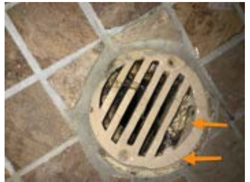
Damaged/Dirty Drain
