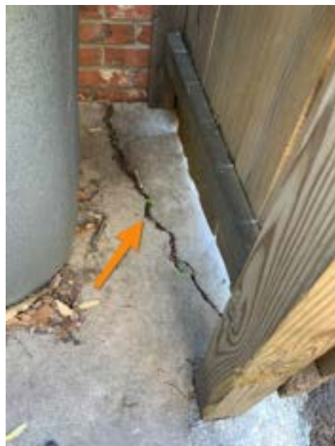
North Gate Walkway
