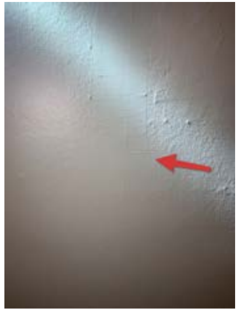
Primary Bedroom-South Wall
