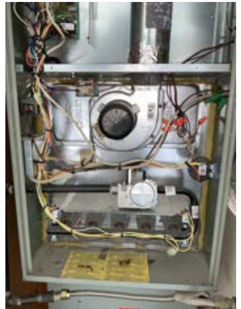
Furnace Manifold
