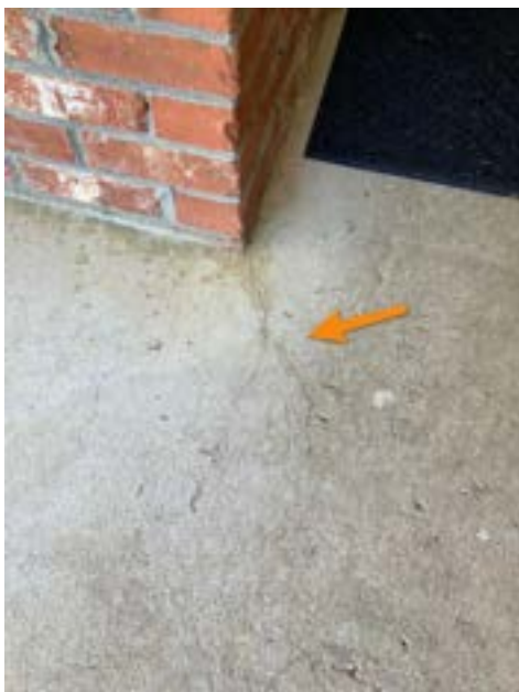
Front Porch Walkway
